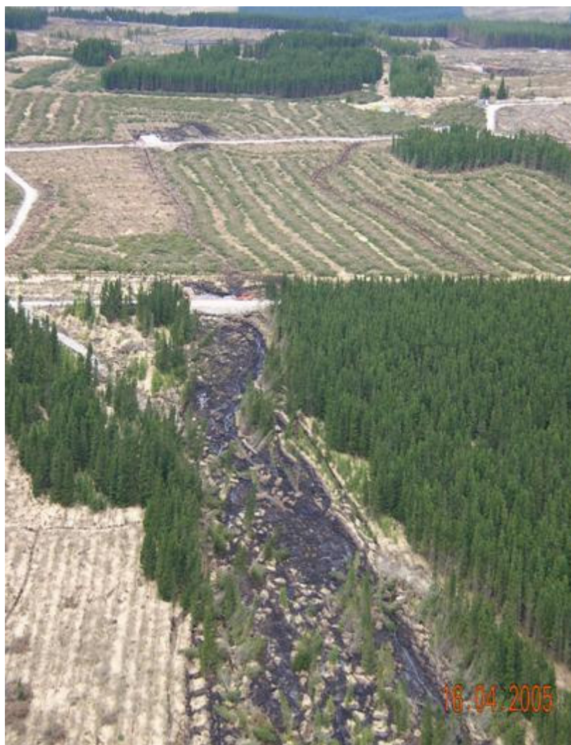
Figure 2.4: Aerial photo of the landslide
