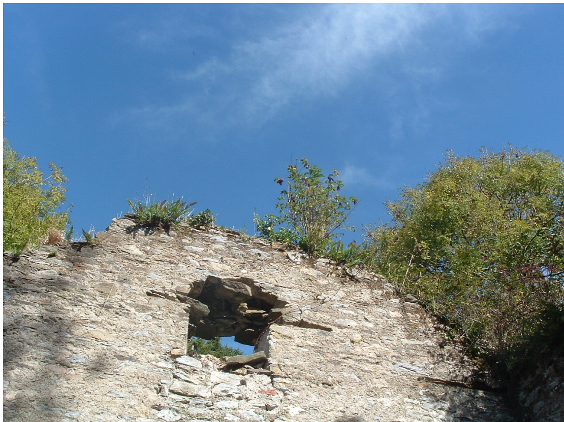
The Corn Mill on site
